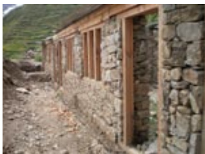
The new extension to Thehe primary school well under way
